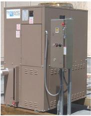
**The Chiller:** The Legacy integrated tank model chiller system is an ideal platform for an Economizer option. These 316SS tank equipped chillers are "closed loop" applications and are Economizer compatible from 1 to 20 tons. Legacy offers both air-cooled and water-cooled condenser configurations. **In Q2 of 2011, Legacy will begin production on its AuraCool retrofit Economizer systems.** The AuraCool system can be deployed on any brand chiller application.
