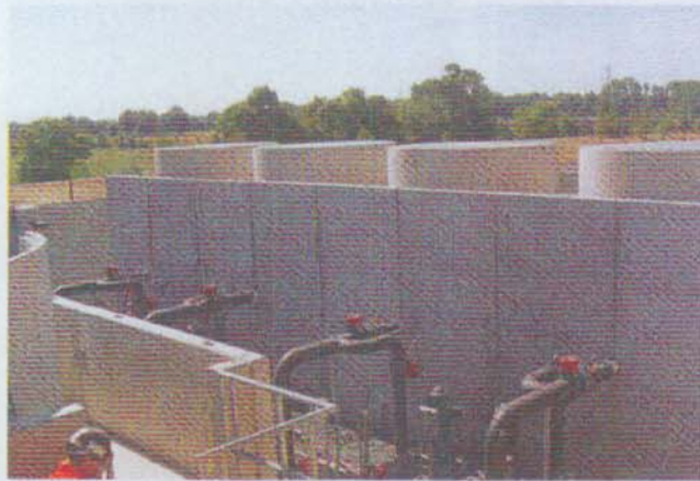
Photo 1: Concrete cooling towers.
