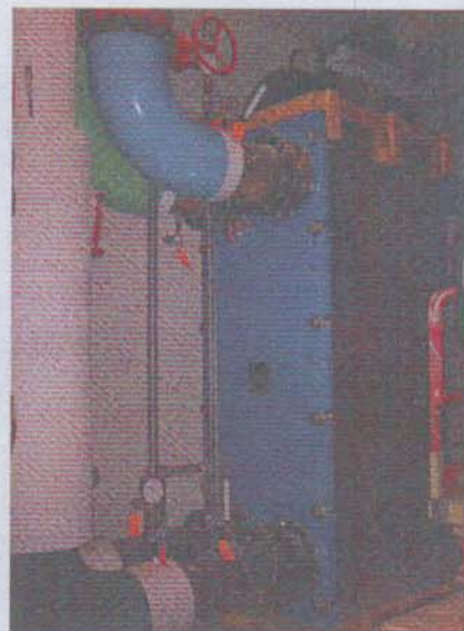
Photo 2: Plate-and-frame heat exchanger.
